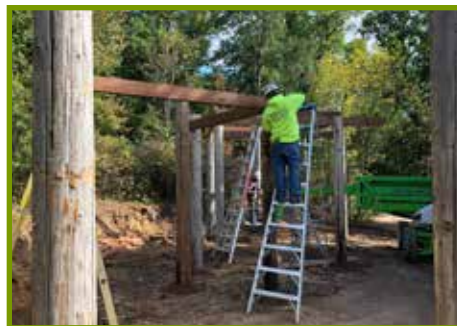
Market & Johnson staff attaching the cross beams. Photo by Staff
