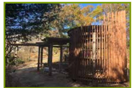
Back view of the rotunda of the Butterfly Pavilion, benches were installed inside for seating. Photo by Adam Fuller of Lien & Peterson Architects
